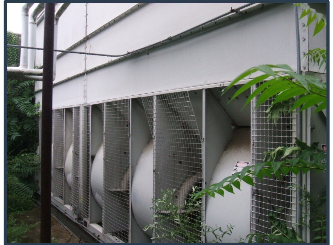
Forced draft type cooling tower – fans blowing thru condenser coils
