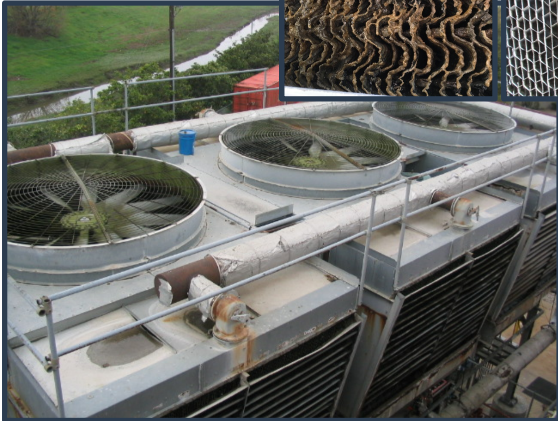
Induced draft type cooling tower – fans drawing air across condenser coils (more common)
