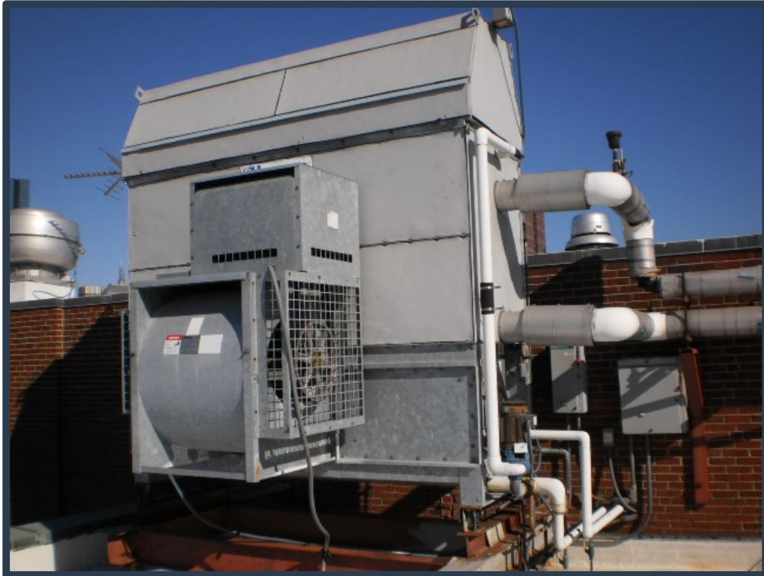
Forced draft type cooling tower – fans blowing thru condenser coils
